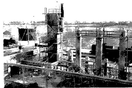
HYGIRTOL plant at Mrs. Tucker's Products, Division of Anderson, Clayton & Co.
